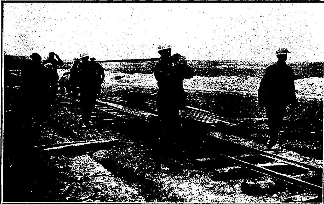
AN INDISPENSABLE ASSET IN THE BRITISH ADVANCE.—Soldiers laying light railways, the use of which have revolutionised transport, ensuring the rapid and safe despatch of necessary war material to the fighting line.
