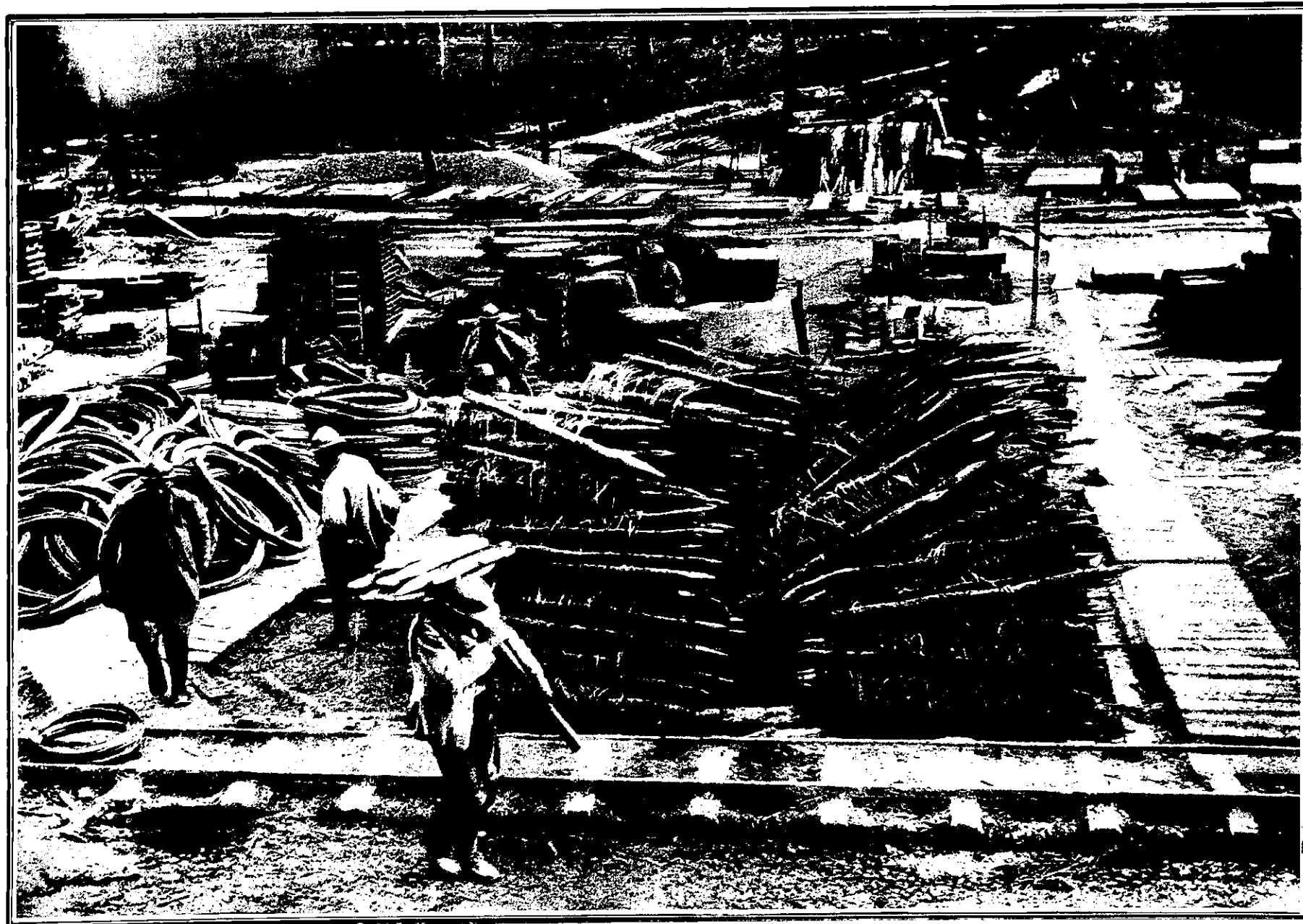
ABUNDANCE OF MATERIAL IN THE FRENCH RESERVE DEPOTS. BARBED WIRE, TELEPHONE AND TELEGRAPH WIRES, STAKES, TIMBERS, DRAIN PIPES, SAND BAGS, CEMENT, AND—LADDERS! A PART OF THE STOCK IN ONE OF THE MANY ABUNDANTLY SUPPLIED RESERVE DEPOTS OF MATERIAL BEHIND THE FIGHTING LINES ON THE FRENCH FRONT.
