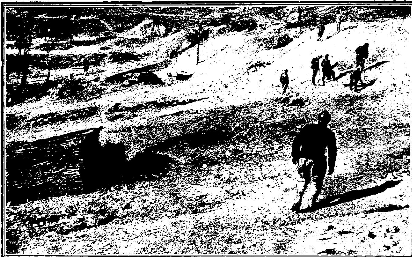
WITH THE FRENCH NORTH OF VERDUN—REPAIRING THE TRENCHES AND UNDERGROUND SHELTERS DURING A LULL IN FIRING OPERATIONS.
