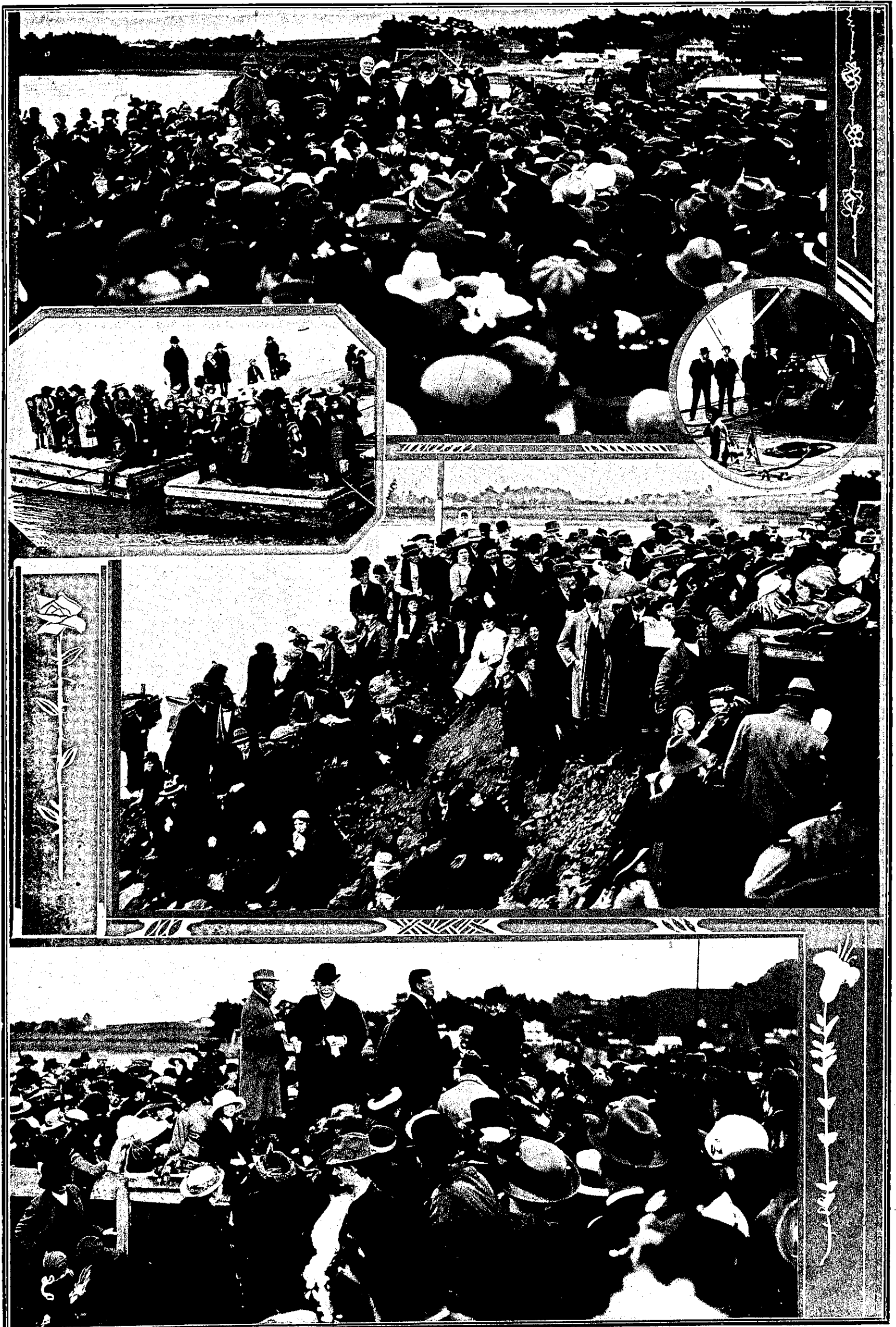
An interesting ceremony was performed by the Prime Minister, Hon. W. F. Massey, on Saturday afternoon, when the first pile was driven in connection with the new bridge which is to span the Manukau between Onehunga and Mangere.
