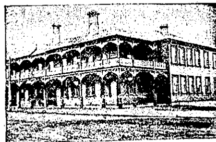
NEW HOTEL (FRONT VIEW)
