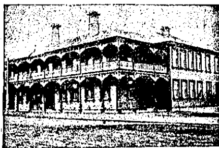
NEW HOTEL (FRONT VIEW)
