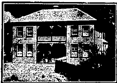
TRAMWAY HOTEL, KARANGAHAKE (Across the Bridge).
