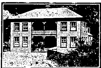
TRAMWAY HOTEL, KARANGAHAKE (Across the Bridge).
