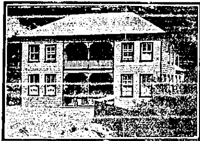
TRAMWAY HOTEL, KARANGAHAKE (Across the Bridge).
