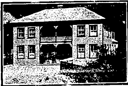
TRAMWAY HOTEL, KARANGAHAKE (Across the Bridge).
