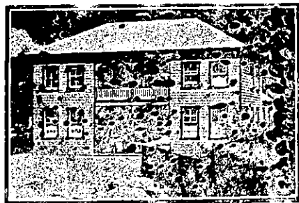
TRAMWAY HOTEL, KARANGAHAKE (Across the Bridge).
