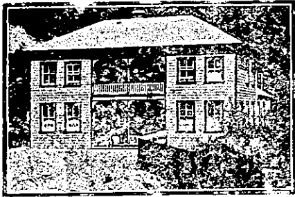
TRAMWAY HOTEL, KARANGAHAKE (Across the Bridge).
