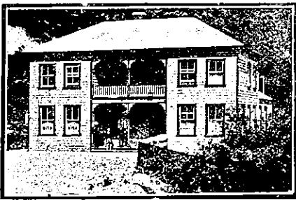
TRAMWAY HOTEL, KARANGAHAKE (Across the Bridge).
