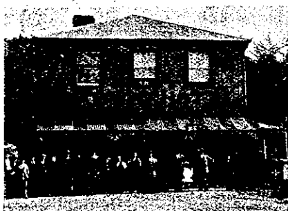
TRAMWAY HOTEL, KARANGHAKE, ACROSS THE BRIDGE.
