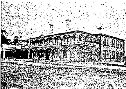
NEW HOTEL, front view.
