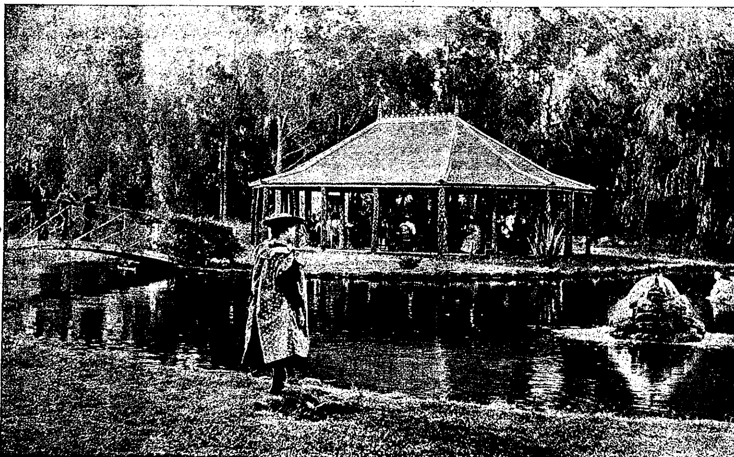
VIEW of LAKE and TEA PAVILLION.
