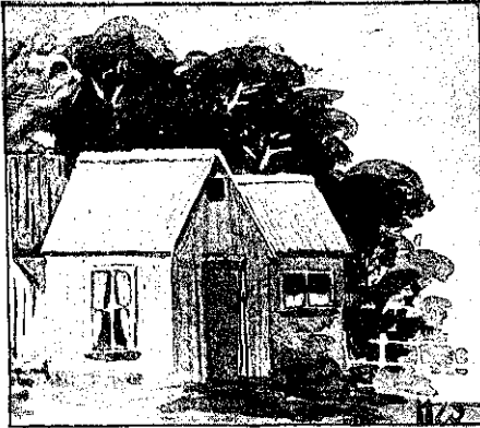
A SETTLER GUMDIGGER'S HOME.
