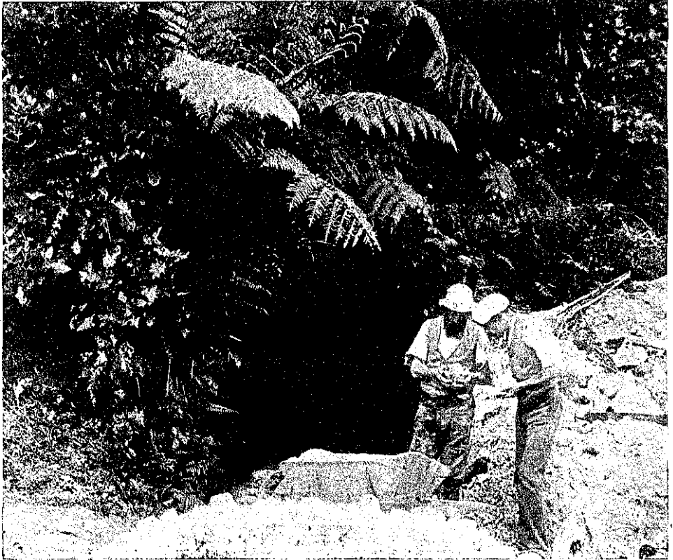
Hes, Photo., HE EMPLOYED HANDS TO PUT IN A DRIVE AND TEST ITS VALUE, Auckland. AND A GOOD FIND WAS THE RESULT.
