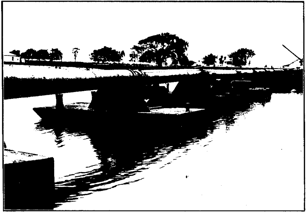
ONE OF THE LINES OF DELIVERY PIPES FOR DISCHARGING DREDGED MATERIAL ON TO THE RIVER BANKS.
