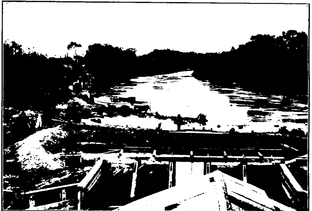
A VIEW SHOWING THE BEND IN THE RANGITAIKI RIVER, FROM WHICH THE NEW OUTLET IS TO BE CUT, AND A TEMPORARY WOODWORK DAM IN THE FOREGROUND.
