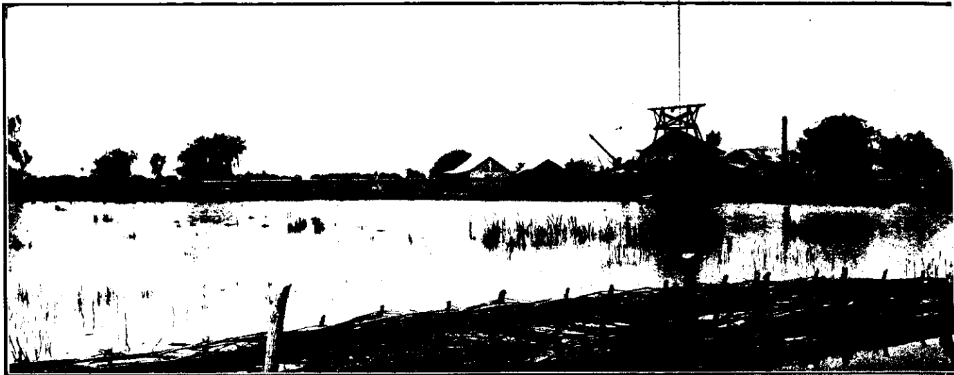
VIEW OF THE SUCTION DREDGE TO BE USED IN CUTTING THE NEW
