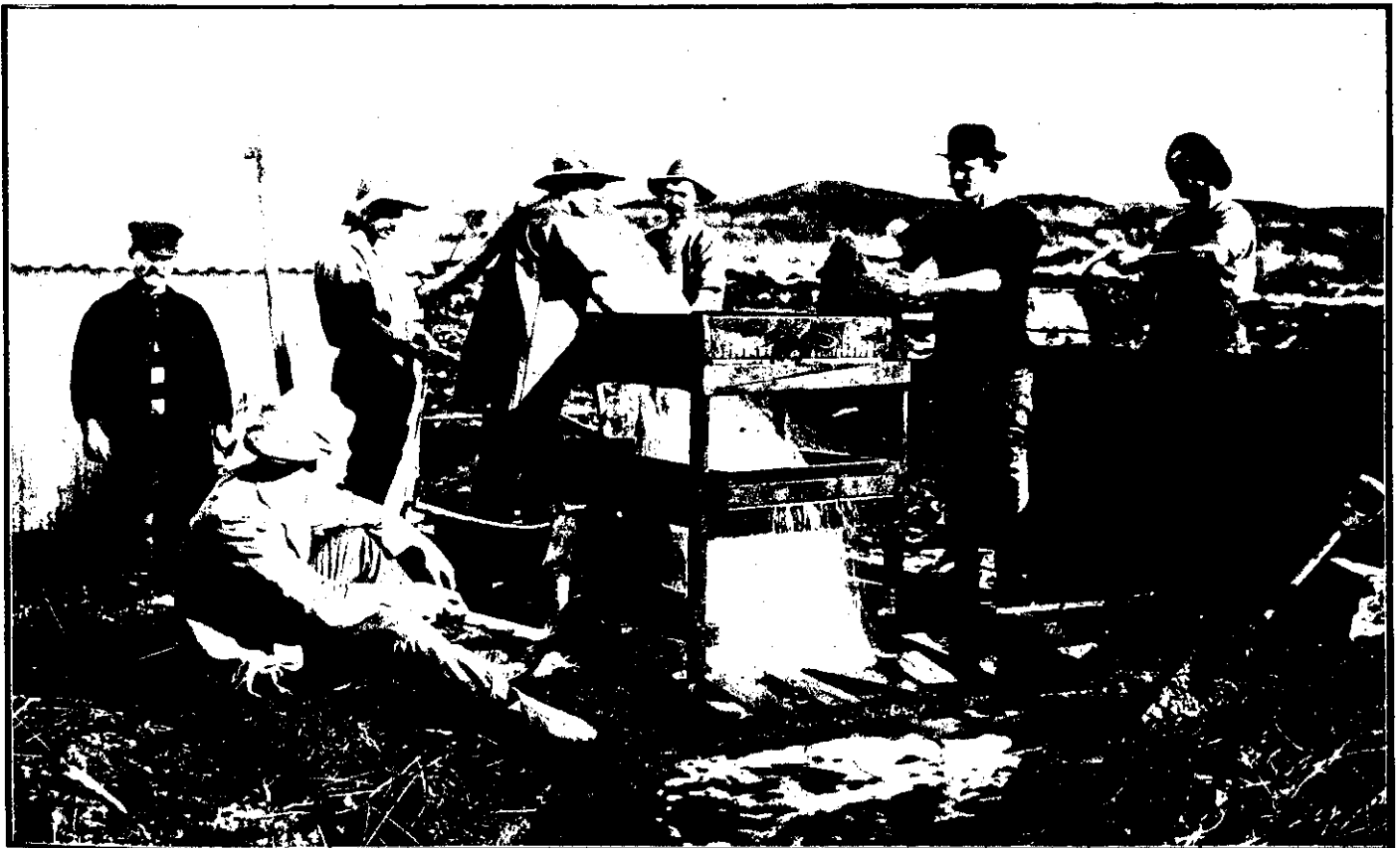
The Austrians in the far North have hit on a far better method of obtaining gum than the ordinary process of digging. They have erected an oil engine and pump, which keeps the "face" of their digging quite dry, and at the same time gives a plentiful supply of water for washing the gum from soil, etc. By this means they are able to work to a depth of eight or ten feet in comfort. The gum and soil are put through a washing sieve, which is kept in motion and very little of any value escapes the keen eye of the Slav. Protected photographs by A. Northwood, Kaitiā.
