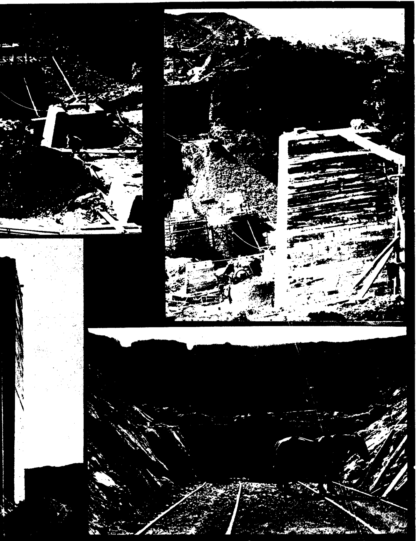
WAVE TO SURMOUNT.—VIADUCTS, CUTTINGS AND EMBANKMENTS IN COURSE OF CONSTRUCTION.
