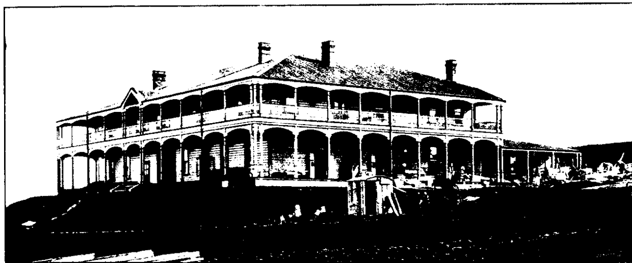
THE PRACTICALLY COMPLETED VETERANS' HOME, AUCKLAND. Taken on the occasion of His Excellency the Governors Final Visit of Inspection last week.
