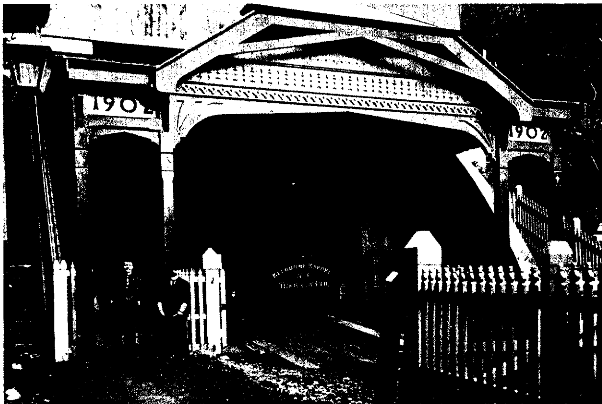
ENTRANCE TO THE KELBOURNE-KARORI TRAM COMPANY'S FIRST TUNNEL, WELLINGTON.
