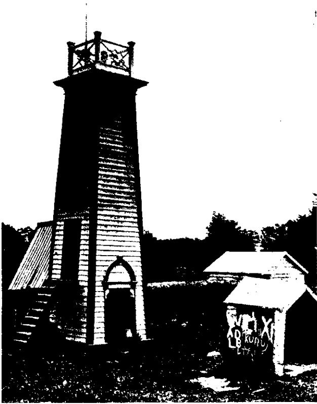
THE WATCH TOWER, formerly used by Armed Constabulary when the Maoris were troublesome.
