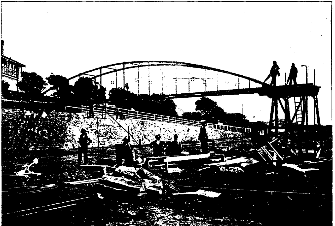
Duroux, photo. STANCHION BRIDGE IN COURSE OF CONSTRUCTION OVER RAILWAY LINE TO ALLOW THE PUBLIC TO CROSS OVER TO THE BEACH.
