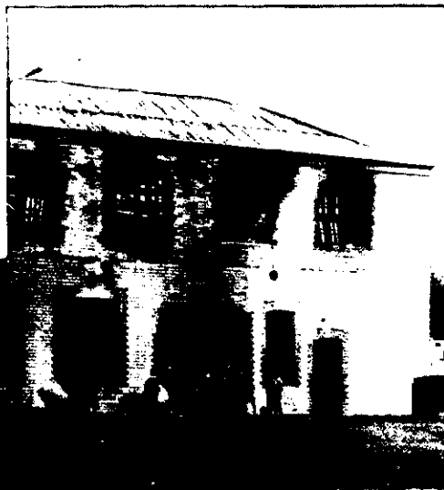
MESSRS. J. D. ROBERTS & CO'S PREMISES, AUCKLAND, DESTROYED BY FIRE LAST WEEK.
