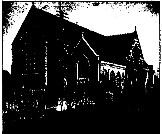
NAPIER CATHEDRAL, showing the new Chapel which is being built in commemoration of peace.
