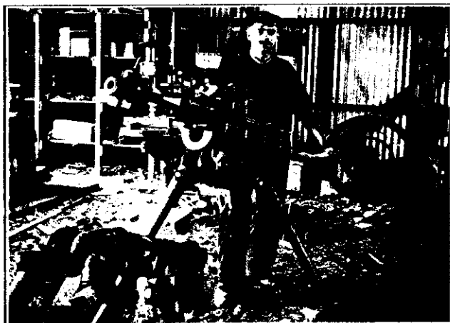
HOW THE COMPRESSED AIR DRILL IS HANDLED.
