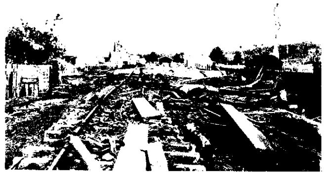
THE RAILWAY STATION YARDS AFTER THE FLOOD.
