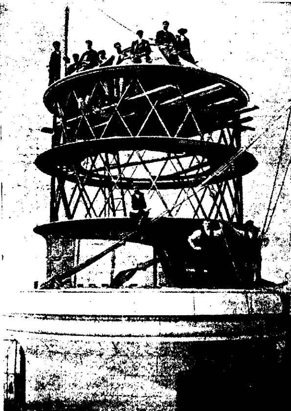
THE NEW LANTERN IN COURSE OF ERECTION.
