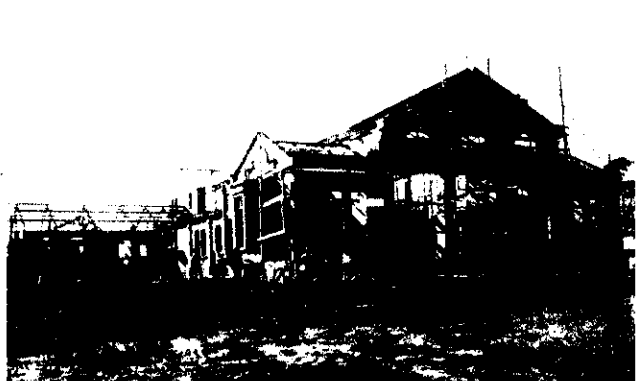
THE TOWN HALL IN COURSE OF CONSTRUCTION.
