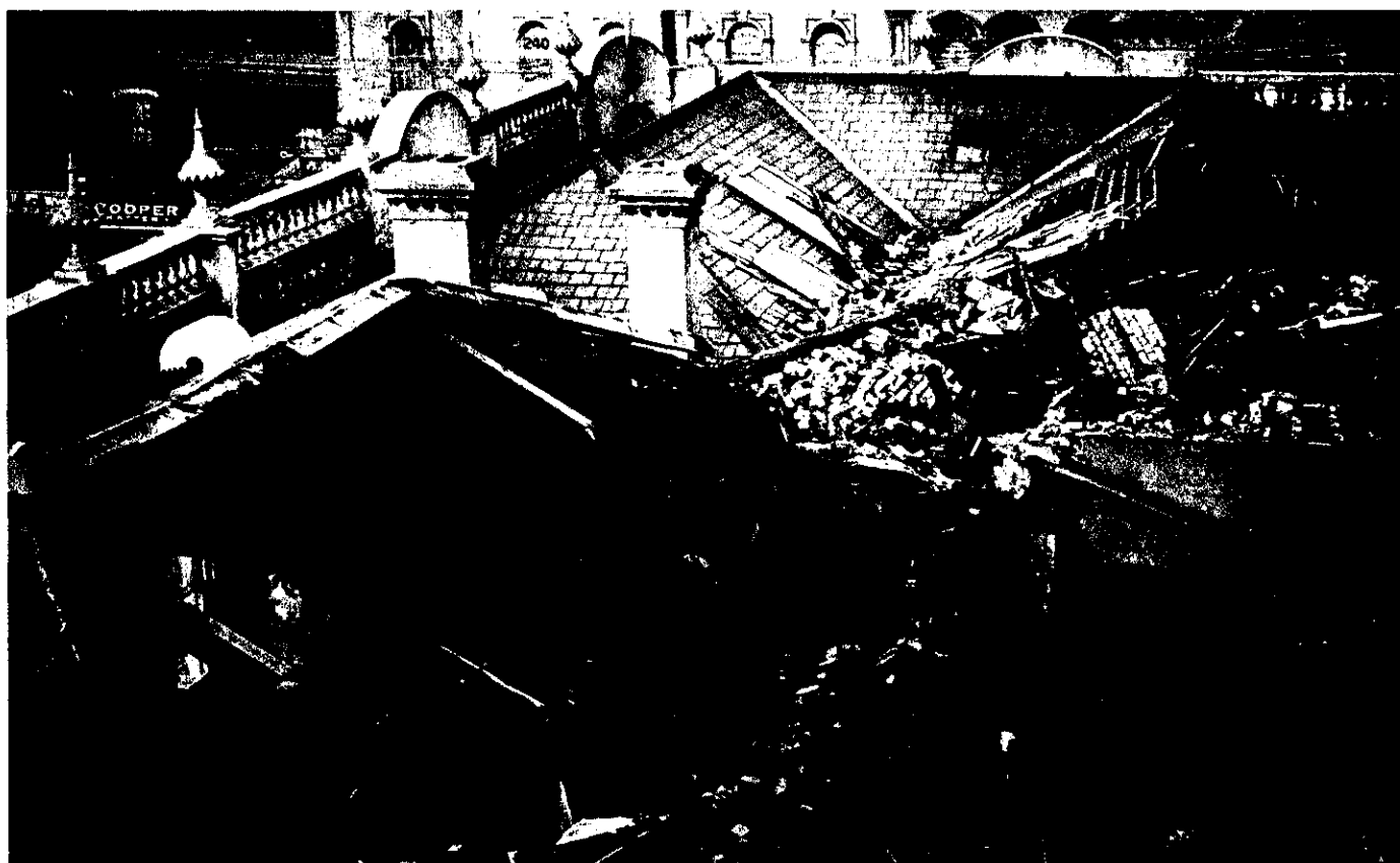
THE THISTLE HOTEL, SHOWING THE DAMAGE CAUSED BY THE FALL OF A WALL DURING THE DESTRUCTION OF THE ARCADE.
