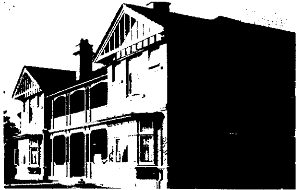
NURSES' QUARTERS AT THE HOSPITAL, OPENED ON SATURDAY BY THE HON. GEO. FOWLDS.
