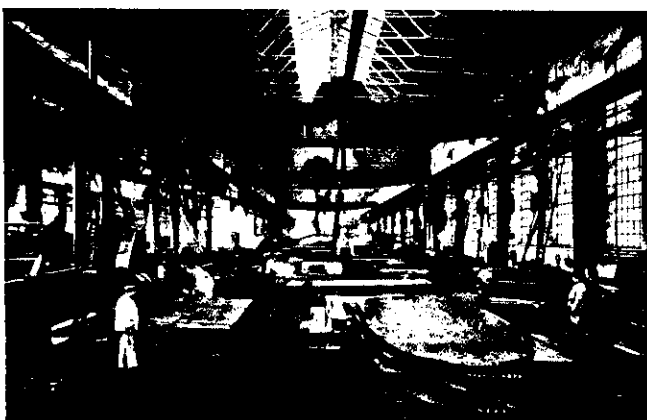
WHERE ARMOUR PLATE IS PLANED.
