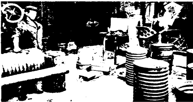
THE COPPER-SMITHS' SHOP AT MESSRS. THOMAS BALLINGER AND CO'S DIXON-STREET WORKS.
