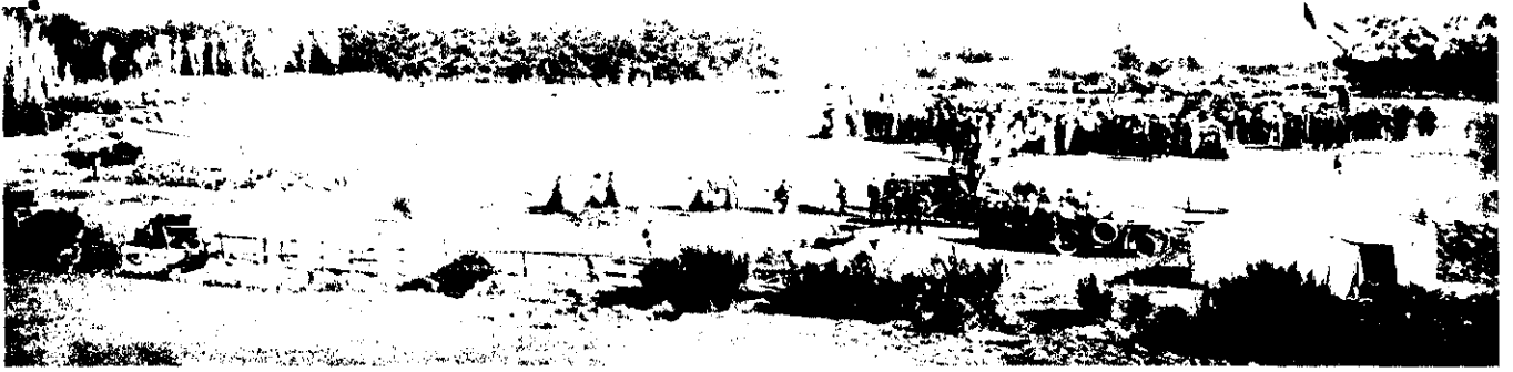
GENERAL VIEW OF THE SITE OF THE NEW BUILDINGS.
