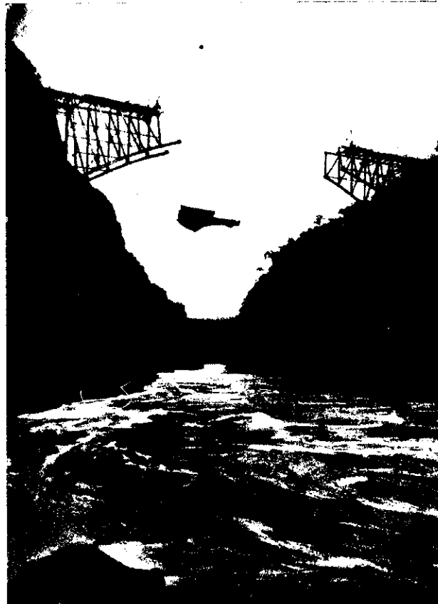
NETS SLUNG TO CATCH FALLING TOOLS OR MEN.
