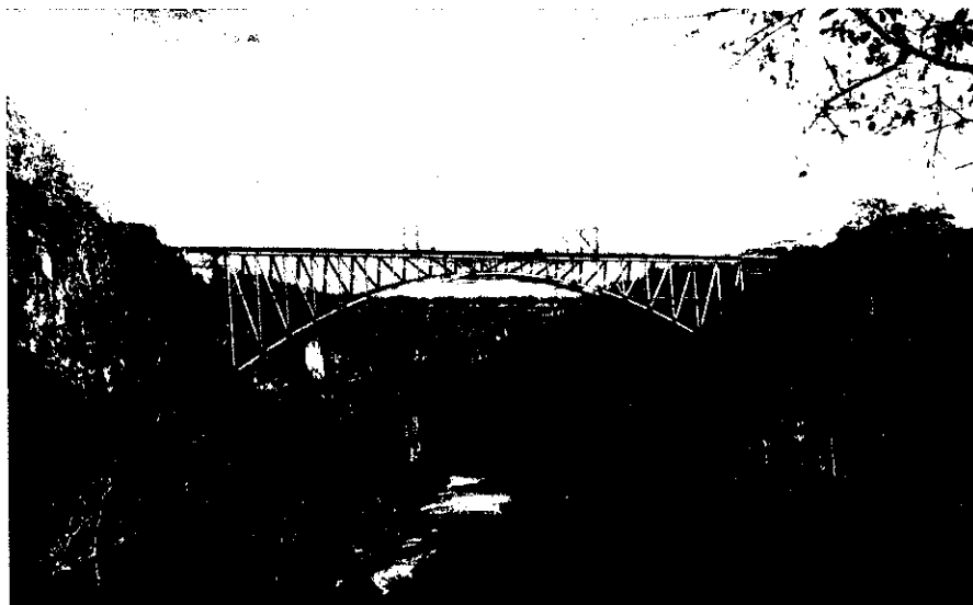
SETTING THE LAST RIVETS IN THE BRIDGE.
