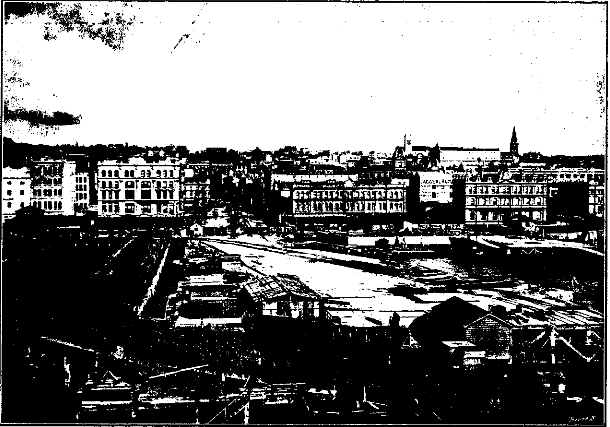
LOOKING UP QUEEN-STREET, FROM AN ELEVATION ON THE QUEEN-STREET WHARF, WHICH IS NOW BEING REBUILT IN FERRO-CONCRETE.
