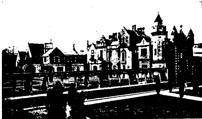
ABBOTSFORD, THE HOME THAT SIR WALTER SCOTT BUILT FOR HIMSELF ON THE BANKS OF THE TWEED.
