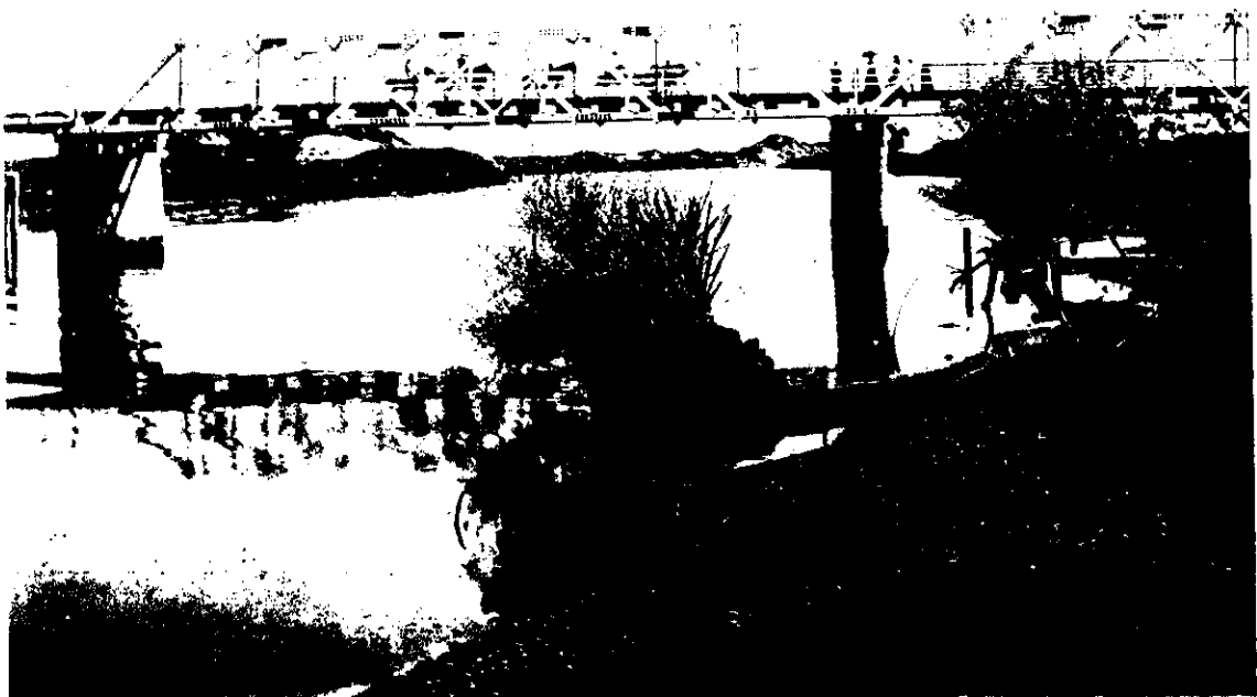
BRIDGE OVER THE MANAWATU, NEAR FOXTON.
