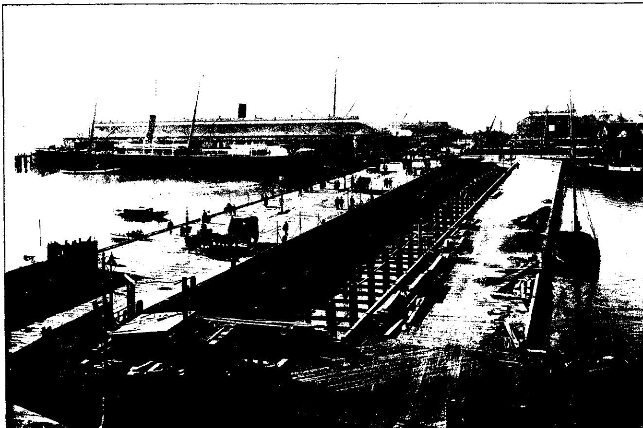
THE PROGRESS OF THE FERRO-CONCRETE WHARF ACCOMMODATION IN AUCKLAND HARBOUR.
