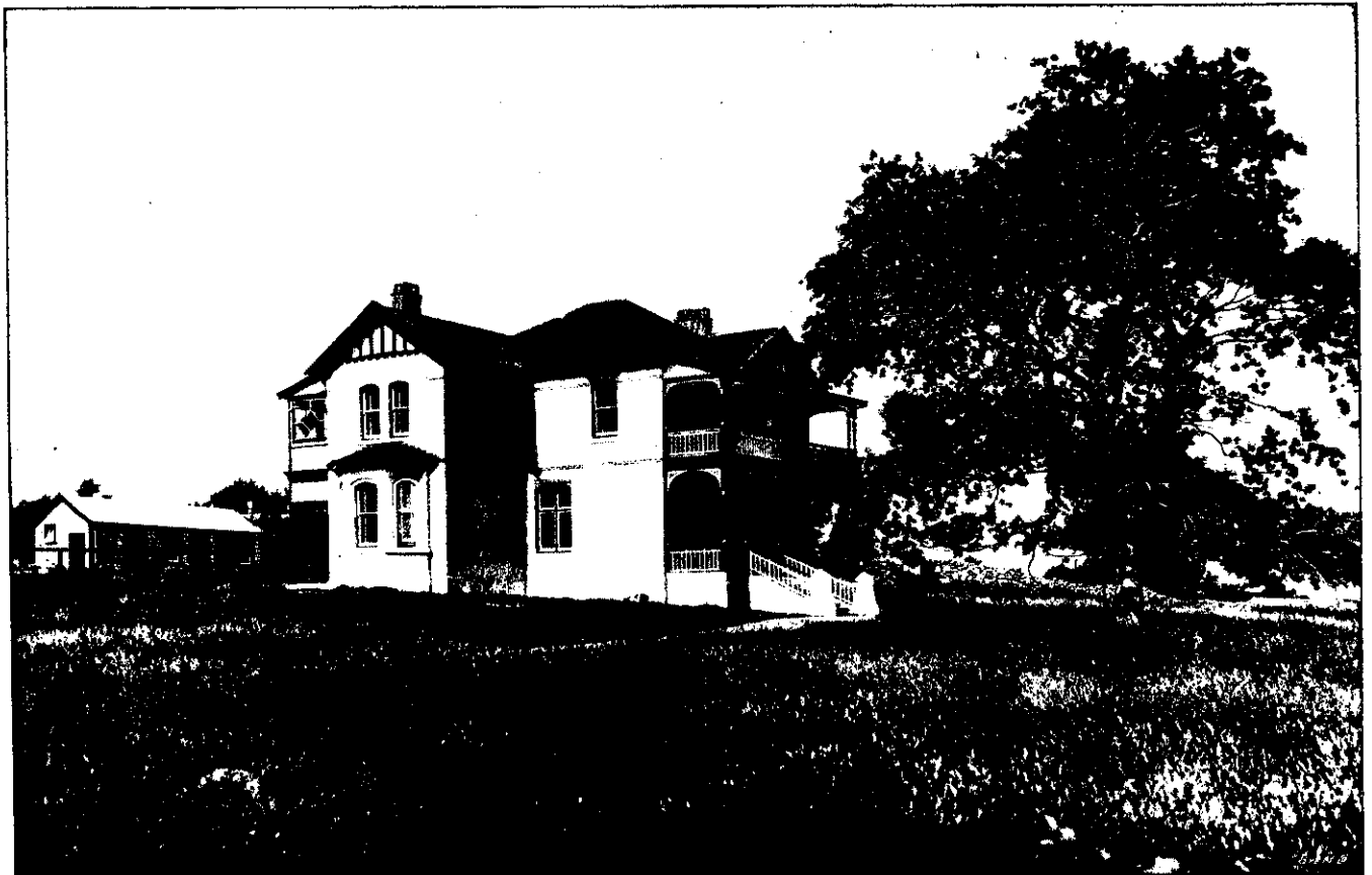
PRESBYTERY OF THE CHURCH OF THE ASSUMPTION, WHICH HAS JUST BEEN COMPLETED.
