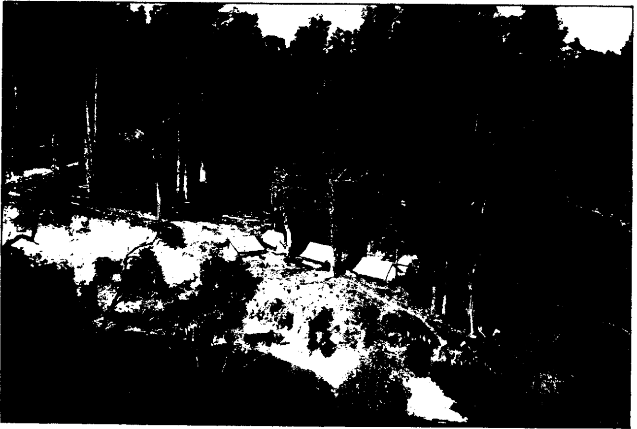
RAILWAY WORKMAN'S CAMP ON THE MAIN TRUNK LINE.
