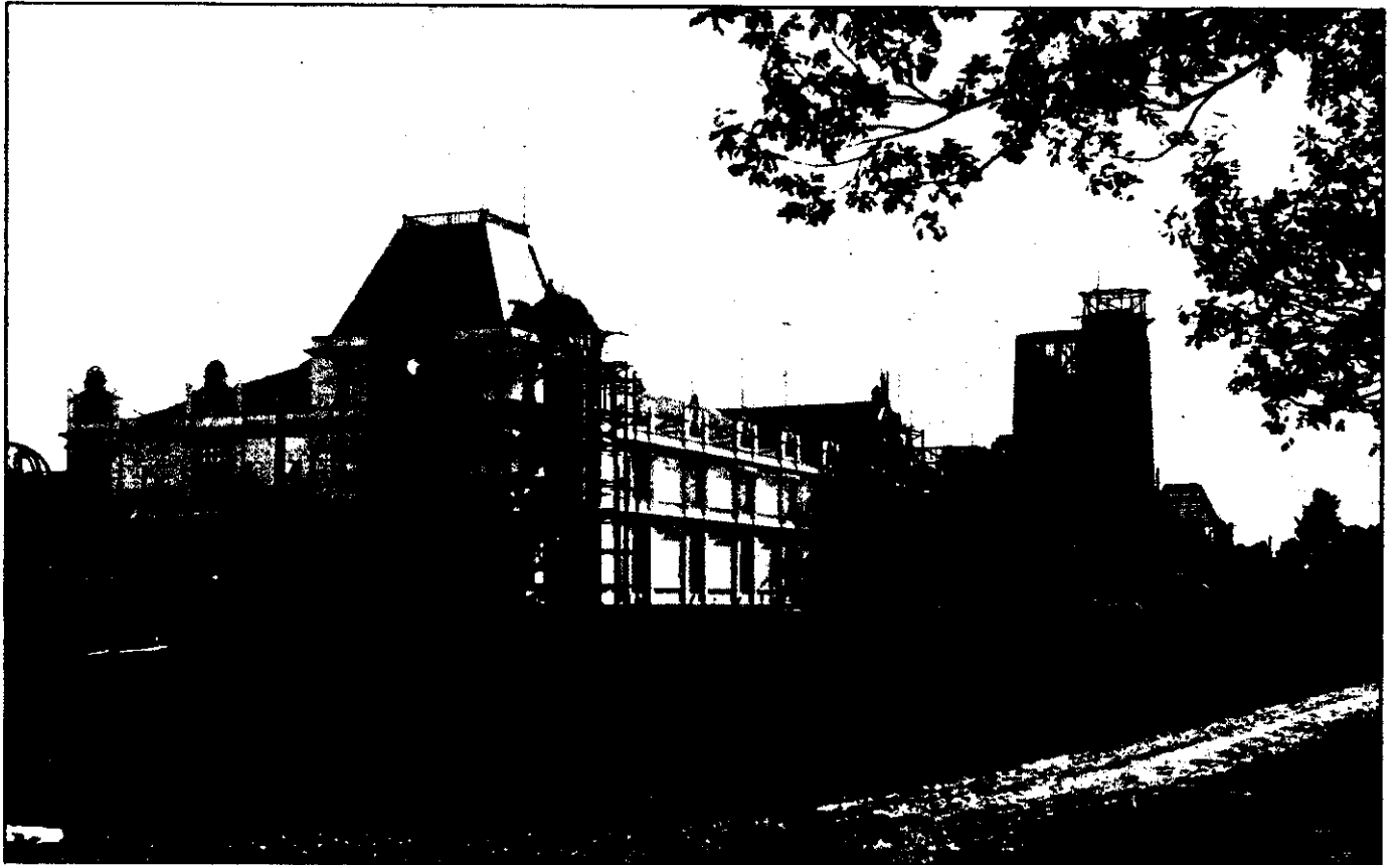
A VIEW OF THE CHRISTCHURCH EXHIBITION BUILDINGS, SHOWING THE PRESENT ADVANCED CONDITION OF THE WORKS.
