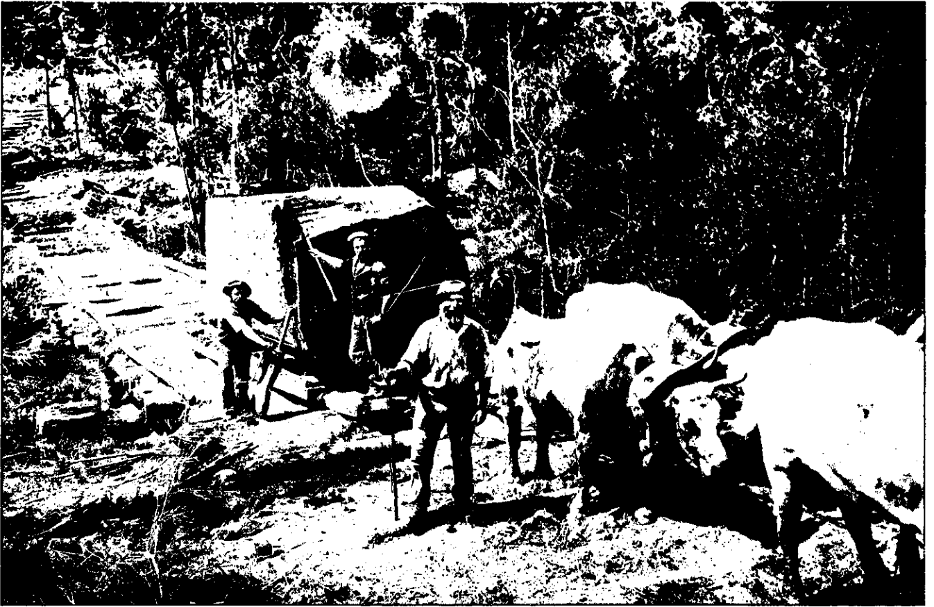
A VAST KAURI LOG, 30 FEET LONG BY 33 IN GIRTH, WHICH HAD TO BE CUT IN HALF AS SHOWN BEFORE IT COULD BE TAKEN ON THE TRAMWAY IN MCCARROLL'S BUSH.
