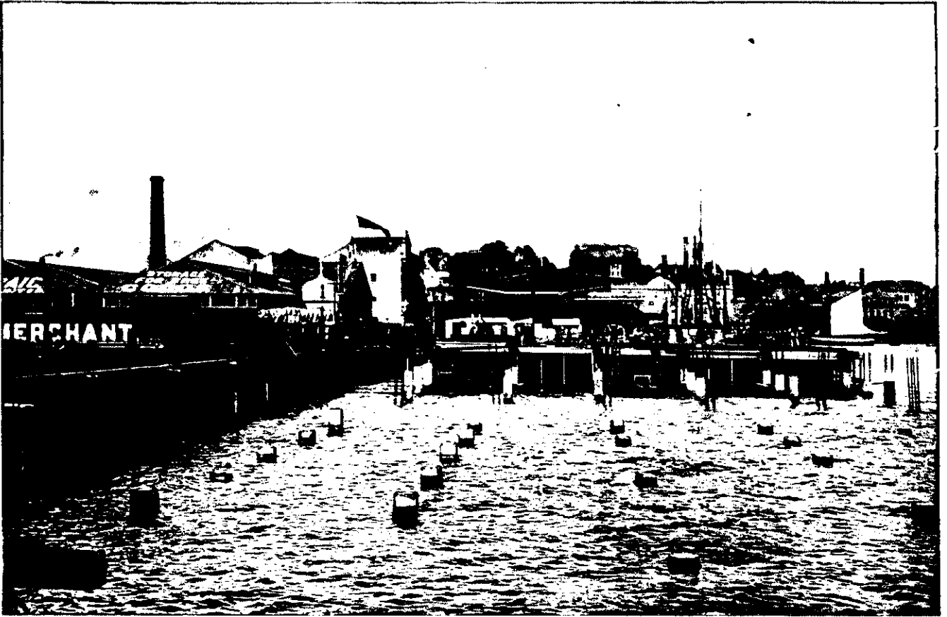
GENERAL VIEW OF THE NEW WORKS.
