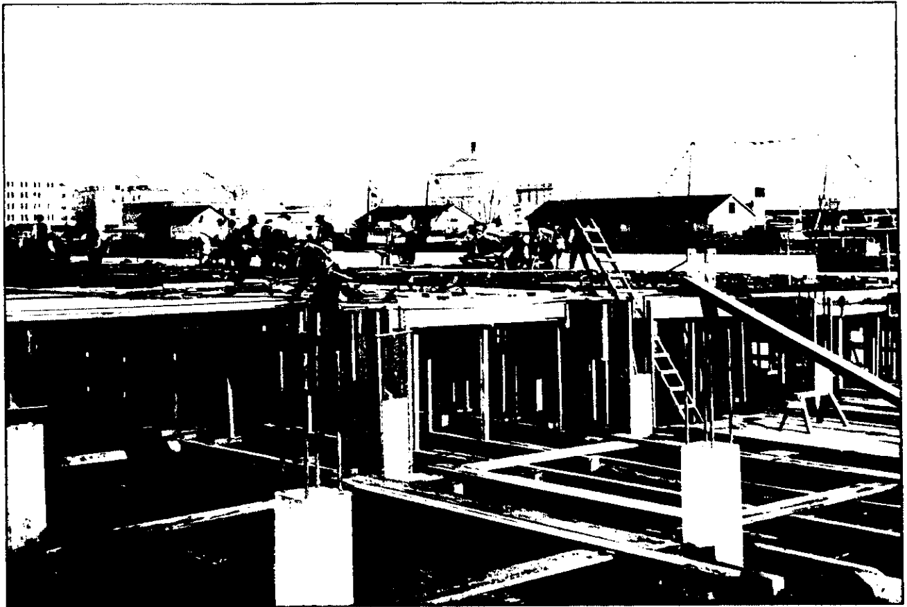
DETAILED VIEW OF THE FERROCONCRETE WORKS AT THE NEW RAILWAY WHARF. Part of Mr. Hamer's big scheme.
