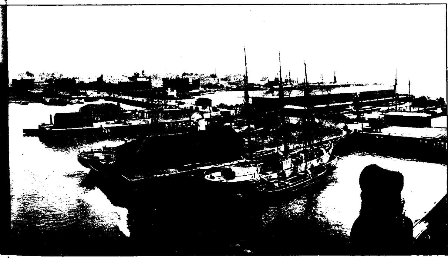
WHARVES AND WATER FRONTAGE.
