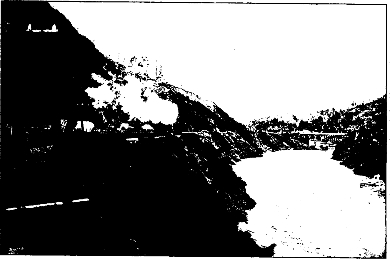
GLIMPSE SHOWING THE TRAFFIC BRIDGE.
