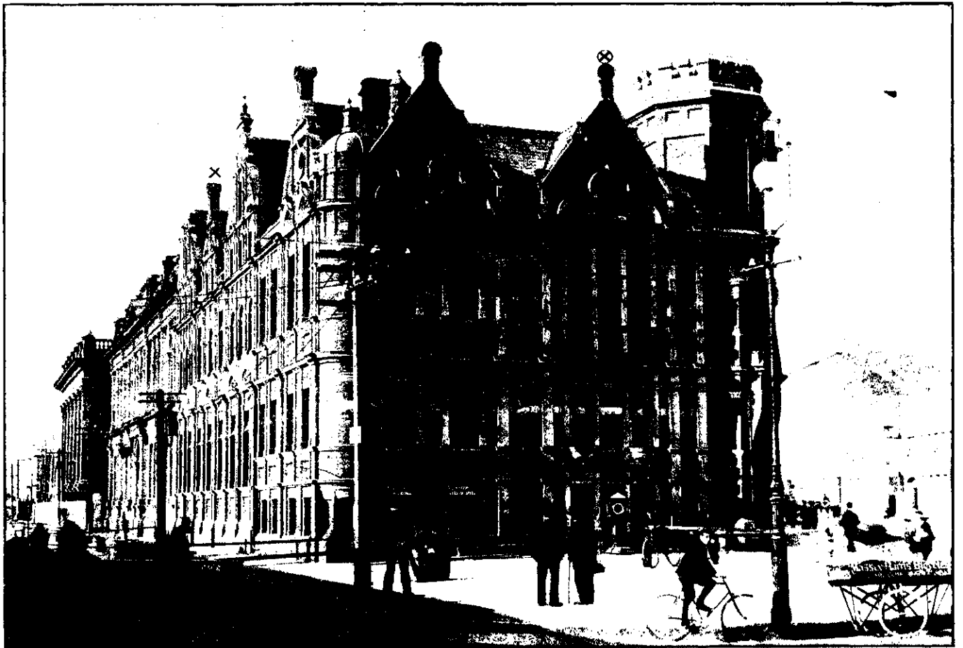
THE PUBLIC LIBRARY. THE SPOTS MARKED ON THE ROOF WERE CONSIDERABLY DAMAGED.
