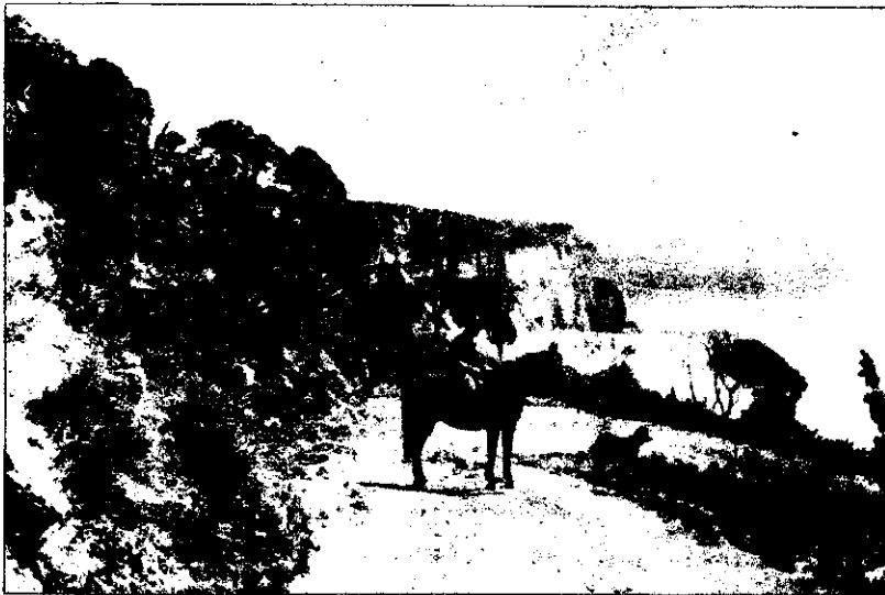
Port Cutting looking North.
