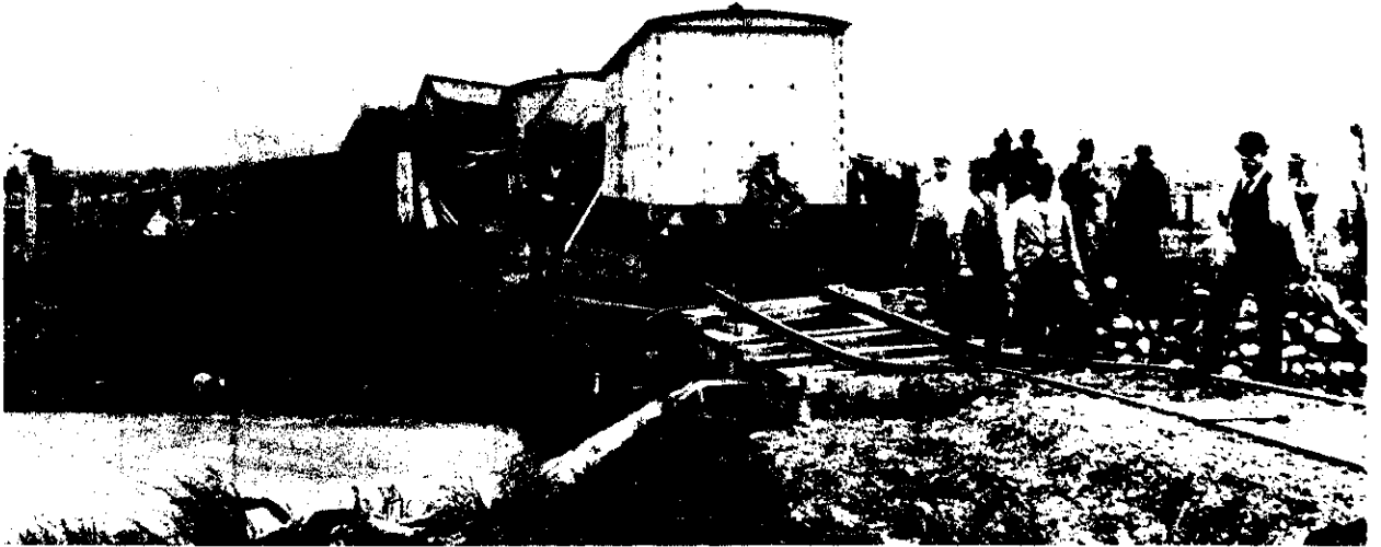
THE SUNKEN BRIDGE: THE CAUSE OF THE ACCIDENT.
