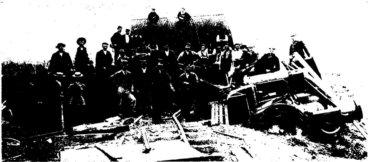
THE DERAILED ENGINE. SHOWING THE DRIVERS IN THE FOREGROUND.
