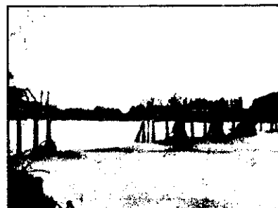
REDCLIFFE BRIDGE, TARADALE.
