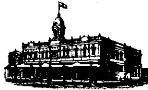
Te Aro House WELLINGTON
